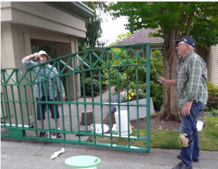
Phil Smith and Lloyd Anderson working on the east gate.
